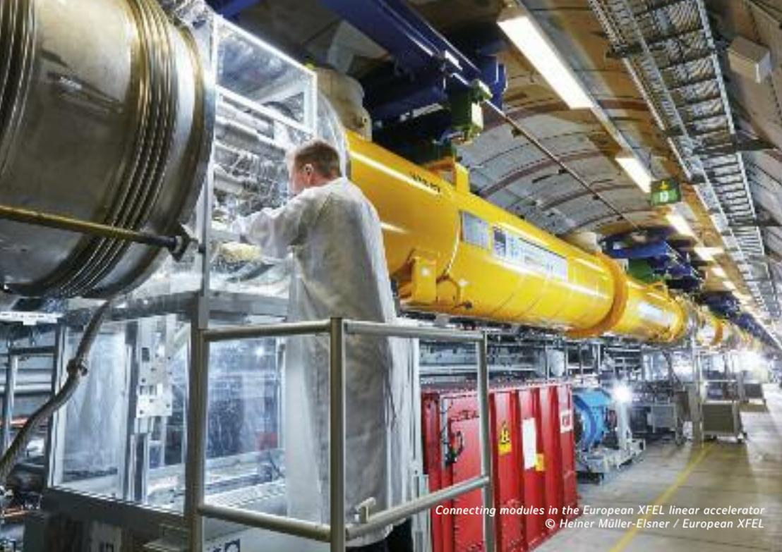
Connecting modules in the European XFEL linear accelerator
